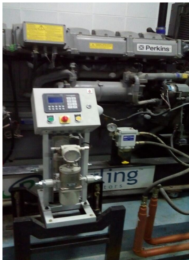
Fig. Installation of FCM on 2000 kVA Perkins Engine, Infosys E-City Bangalore Campus
