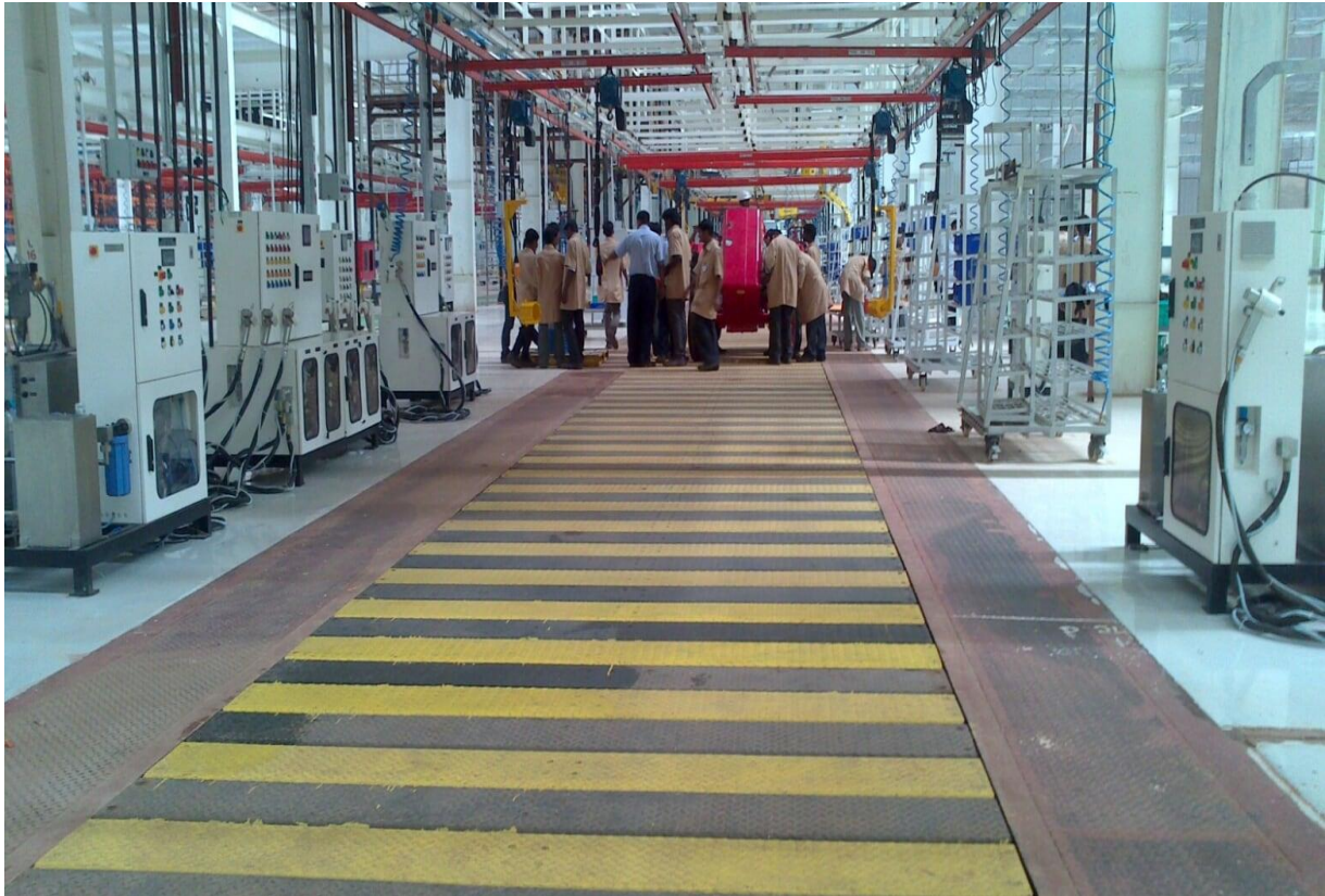
Fig. Turnkey Project of Liquid Management System at M&M Zaheerabad Plant
